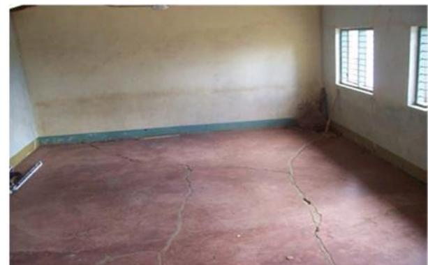
**Figure 8** Heaving of interior floor causing cracking of slab
