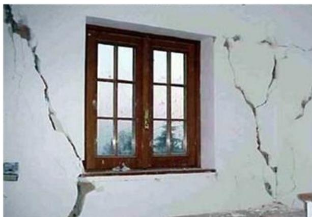
**Figure 6** Serious cracks around window in the interior wall
