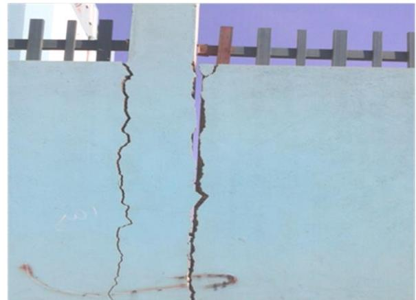
**Figure 3** Sever vertical cracks appeared at the joint between column and masonry wall of the fence
