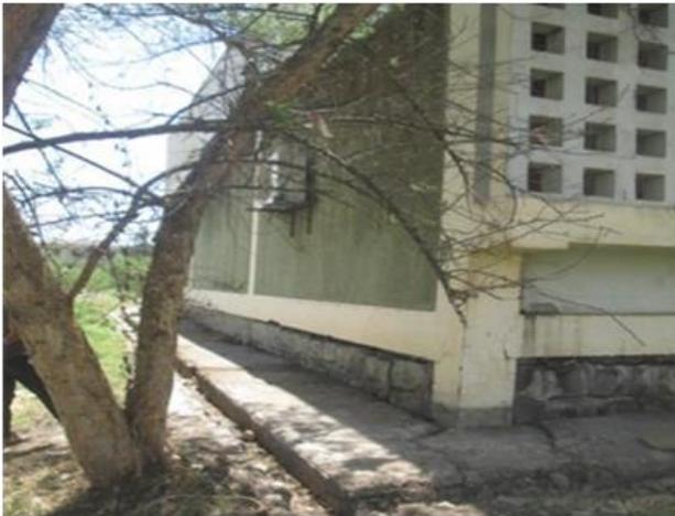
**Figure 5** Foundation wall partially settled around the corner due to trees nearby the building
