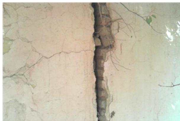
**Figure 4** Severe and deep cracks appear in the exterior walls of the building
