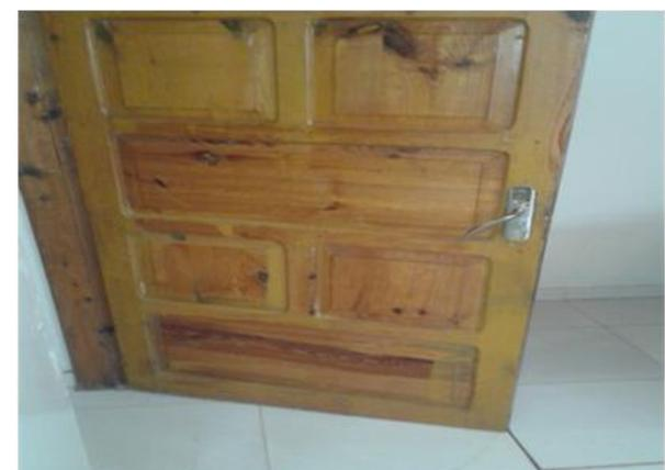
**Figure 9** Doors not properly close or open due to movement of floor
