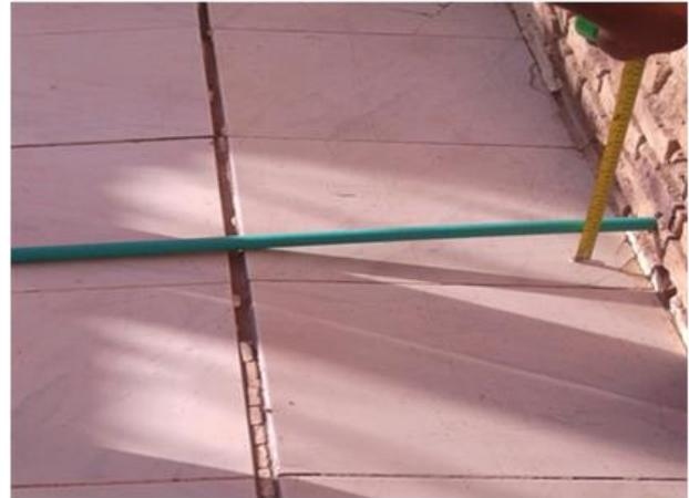
**Figure 7** Floor heave resulted in considerable difference in level about 5.5 cm
