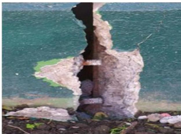
**Figure 10** Severe cracking in concrete perimeter wall showing exposed reinforcing
