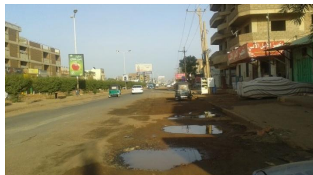
Plate 6. Severe failures of road edges due to water ponding on surface.
